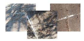
The tennis court surface is cracked and broken and in need of repair. The damage caused by wear and tear and tree roots. The project to fix it required us to remove the three redgum trees that were growing within the fence-line right next to the tennis court. We expect the new synthetic grass tennis court surface will be laid around the middle of the year.
